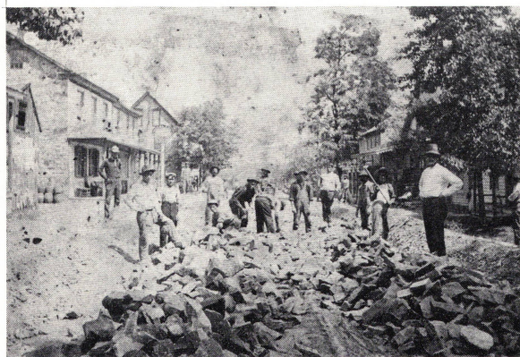
LAYING OF ROUTE 443
