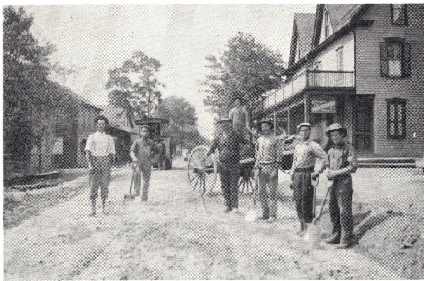
LAYING OF ROUTE 443
