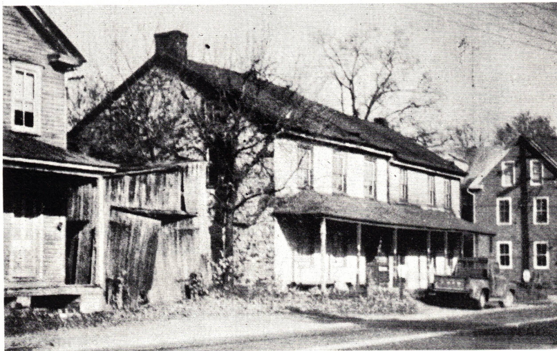
Former Keller's Hotel and Garages.
